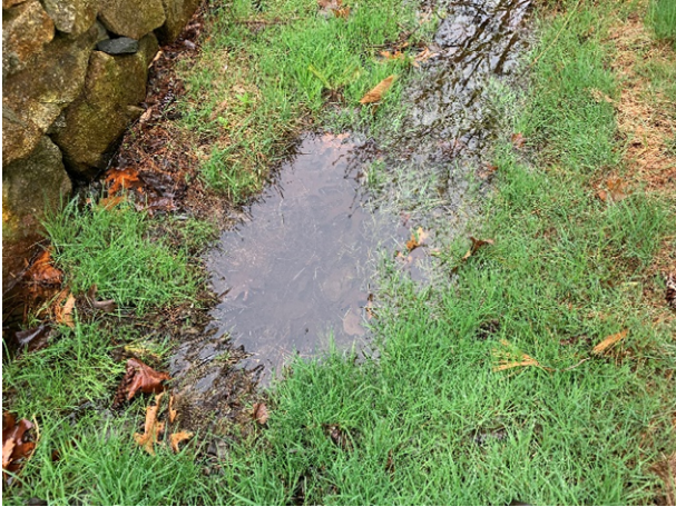
4 Brickyard Circle – 3 (Drainage Course)
