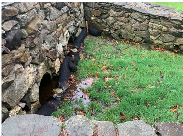
4 Brickyard Circle - 1 (Drainage Course)
