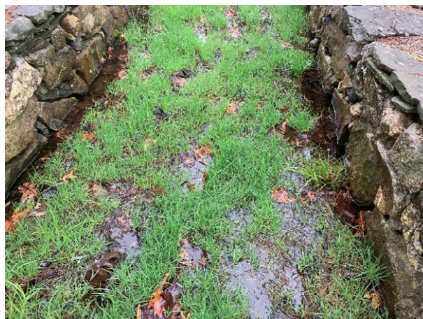
4 Brickyard Circle - 2 (Drainage Course)
