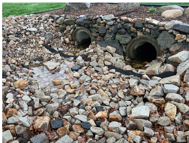
64 Gundalow - 2 (Drainage Course)
