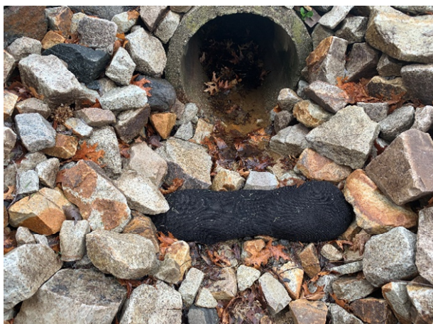
64 Gundalow - 1 (Drainage Course)
