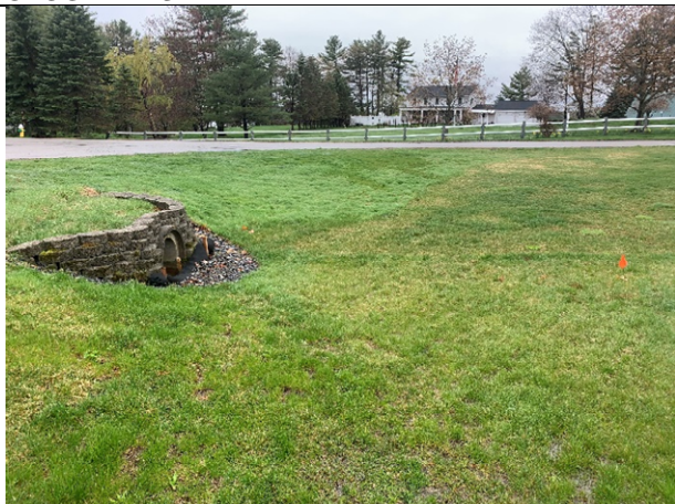
29 Gundalow - 1 (Drainage Area)
